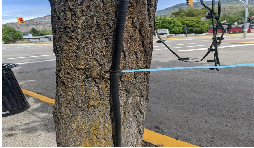
Tree is beginning to grow around the conduit.
